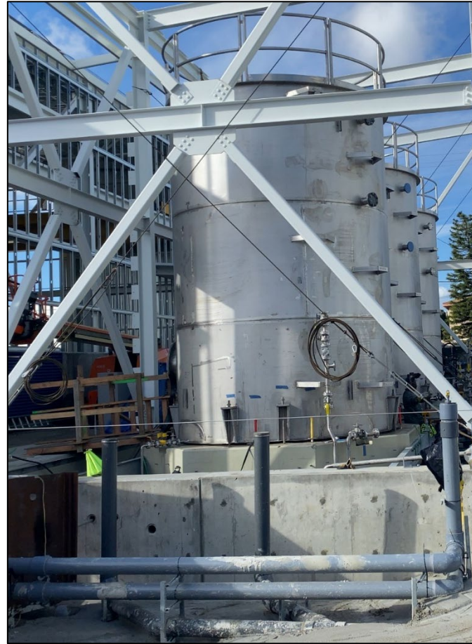
Hydrogen Peroxide Tanks
